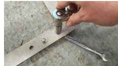
M10x80mm Studs 8.8 HT BZP fixed to Jig rests on mesh
