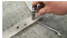
M10x80mm Studs 8.8 HT BZP fixed to Jig rests on mesh
